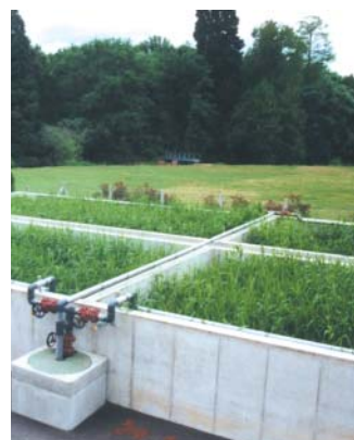
Station de Ligny-le-Ribault, Loiret
