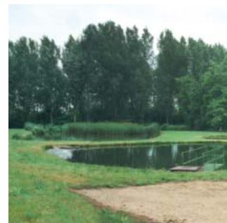
Station lagunage, Cour-sur-Loire
